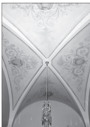
Restored ceiling in S-224
